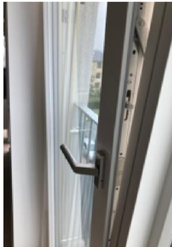
Half open. Press on the door and move the handle into a horizontal position.
