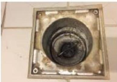
**Step 3: now you can reach the water trap which stays deeper in the drain**
