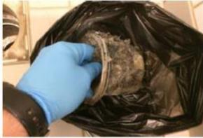
**Step 6: place the water trap bowl in a nylon bag. Remove the built-up hairs and put them in the nylon bag (it is not allowed to put the flith in the toilet as it can cause further blockage!)**
