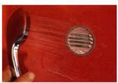
Step 8: put everything back firmly to its place and fill the water trap up with water in order to stop the smell.
