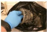
Step 6: place the water trap bowl in a nylon bag. Remove the built-up hairs and put them in the nylon bag (it is not allowed to put the flith in the toilet as it can cause further blockage!)
