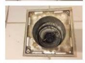
Step 3: now you can reach the water trap which stays deeper in the drain
