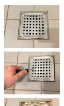
Step 1: remove or loosen the 2 screws in the corner of the grid (some grids have no screws)
