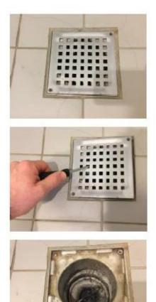
Step 1: remove or loosen the 2 screws in the corner of the grid (some grids have no screws)
