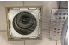
Step 8: place the water trap well in its place and fill it up with water in order to stop the drain smell. Finally place the grid back.
