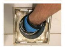
Step 1: remove or loosen the 2 screws in the corner of the grid (some grids have no screws)
