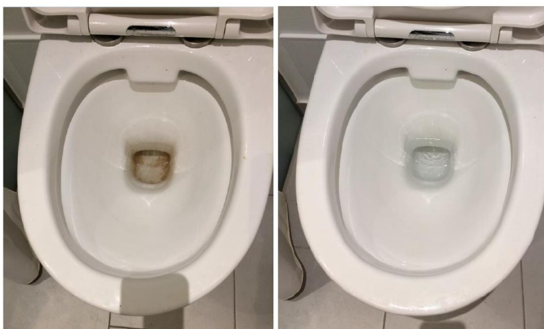
Example of how regular cleaning using only a toilet brush can prevent build-up.
