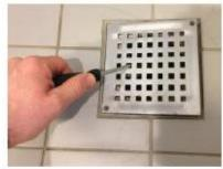
Step 2: lift the grid up and remove it to reach the water trap
