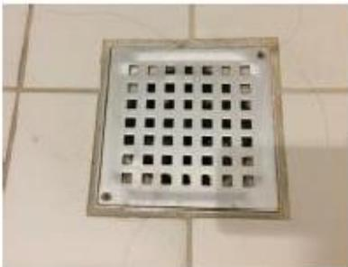
**Step 1: remove or loosen the 2 screws in the corner of the grid (some grids have no screws)**
