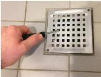
**Step 2: lift the grid up and remove it to reach the water trap**
